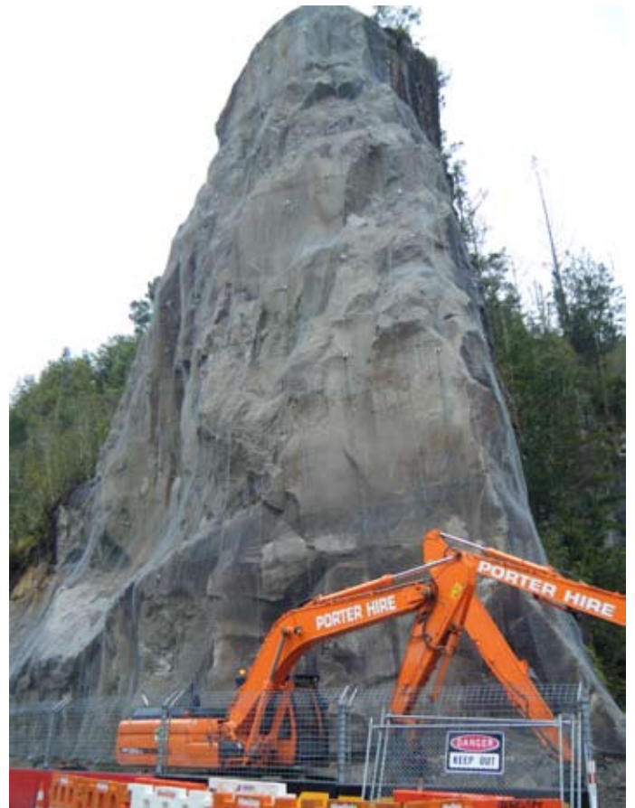
Meshing on the peak nearing completion.
