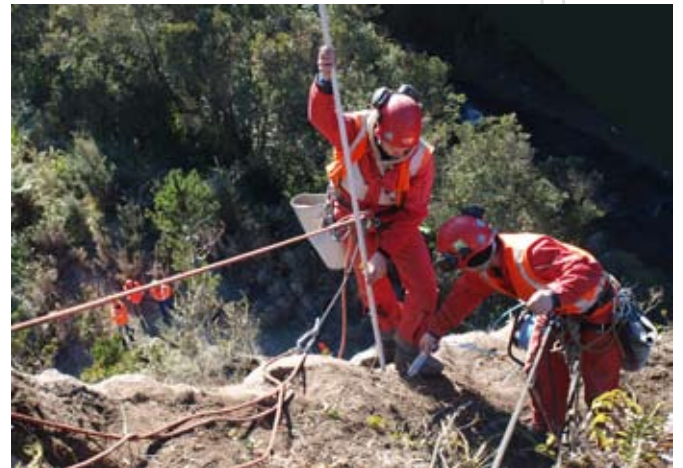
Loading explosives on blast day.
